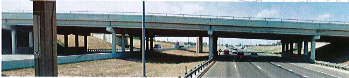
Atypical Bridge Structure: No Column in Median
