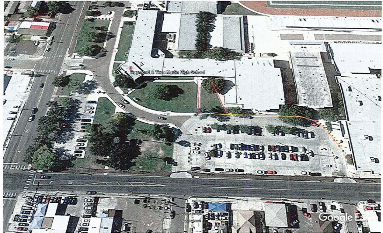
Repairs/re-construction of sidewalks on the east side of main building due to existing damage. 600 Linear feet.
