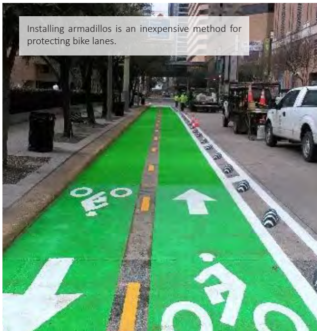
PROTECTED LANE WITH ARMADILLOS IN SAN ANTONIO, TX
